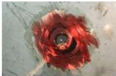
Figure 5. Head spin hole plug weld after the application of the penetrant.
